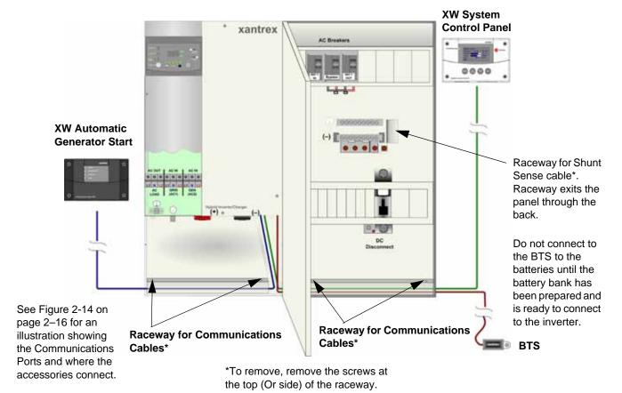
Figure 2-8 Routing Communications Cables
